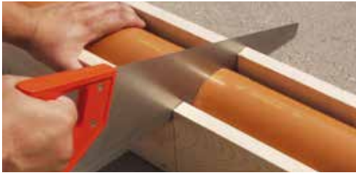
Figure 2 Pipe cutting with a hand-saw
